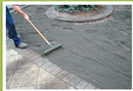
Preparing the 20mm crushed rock
