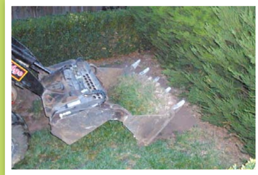
Excavation of area by hand or machine
