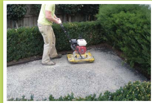
Compacting the base
