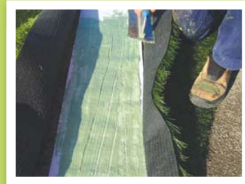
Trowelling adhesive onto seaming tape
