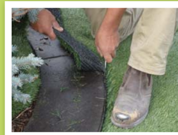
Trimming around edges
