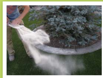
Broadcasting the infill sand
